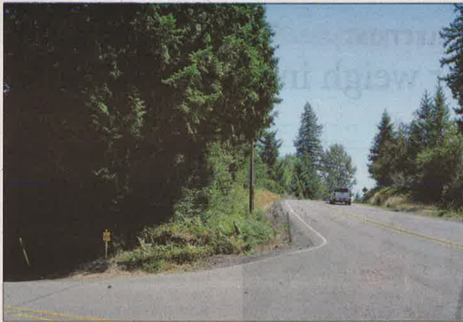
The intersection of state Route 3 and state Route 302 in Belfair will likely need to be modified to accommodate increased truck traffic drawn by the State Route 3 Freight Corridor. The current northbound turn onto state Route 302 is nearly 110 degrees, and the shape of state Route 3 creates a blind corner for traffic trying to turn southbound. Journal photo by Justin Johnson
