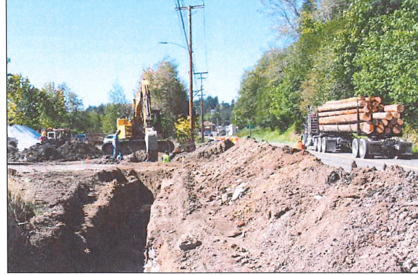
After decades of discussions, the Pear Orchard Park and Ride on state Route 3 near the railroad overpass in Shelton is expected to be completed by the end of the year. Journal photo by Gordon Weeks
